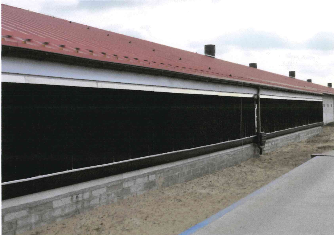
Rys 1. System Pad Cooling
